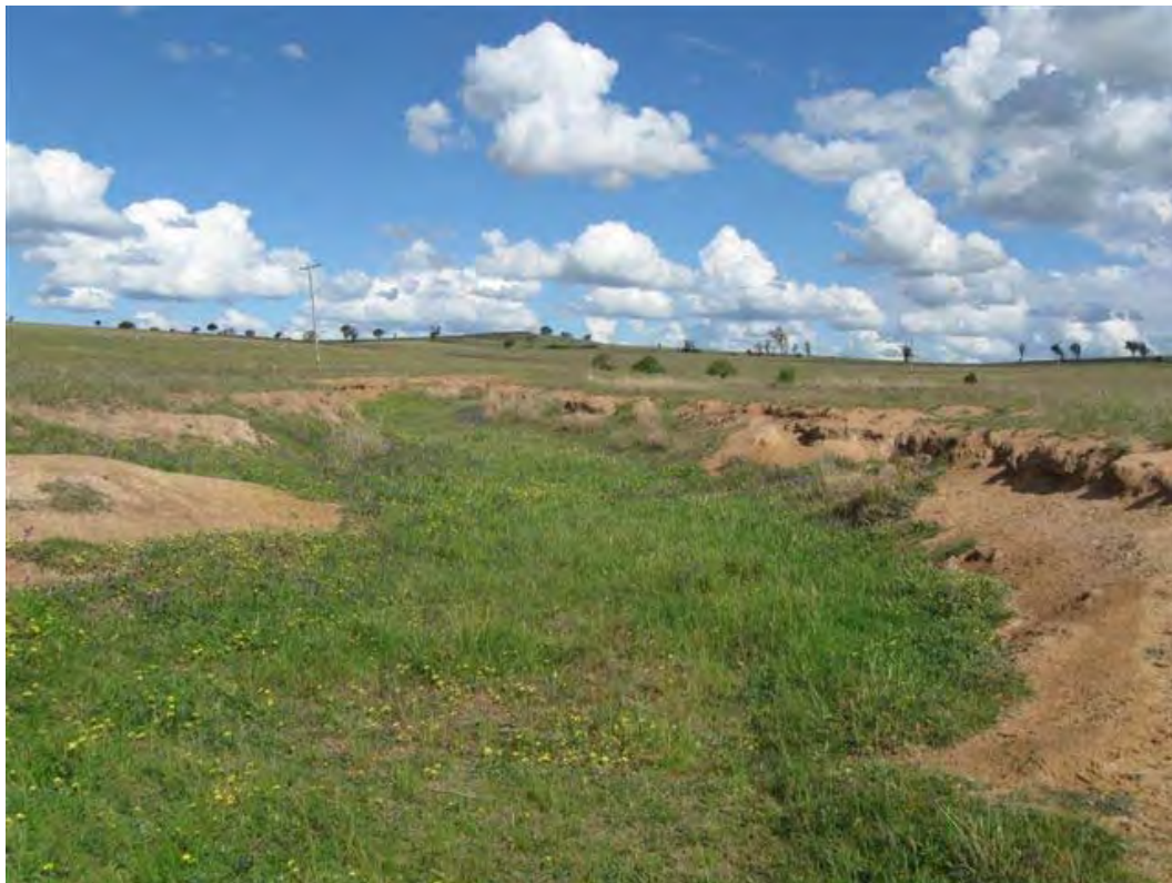
Plate P12: Typical streambank erosion, showing level of exposure on an un-named 2 nd -order drainage line east of Junee, Transect 7
