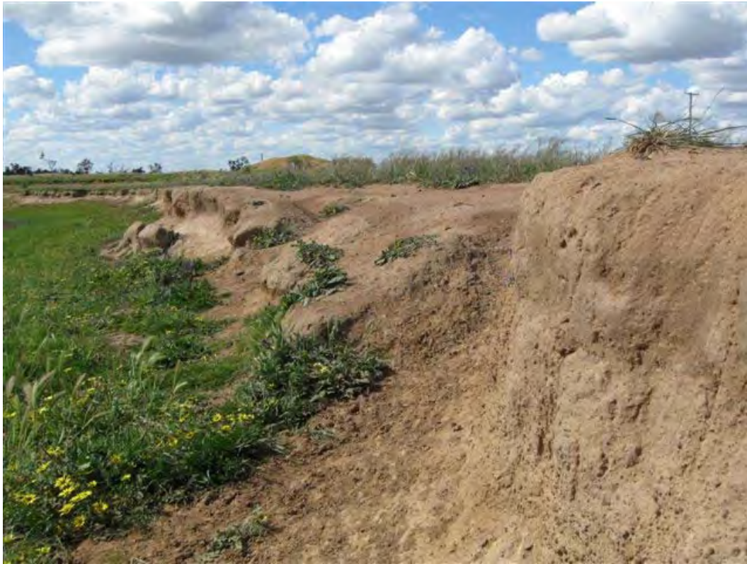
Plate P13: Streambank erosion east of Junee, Transect 7
