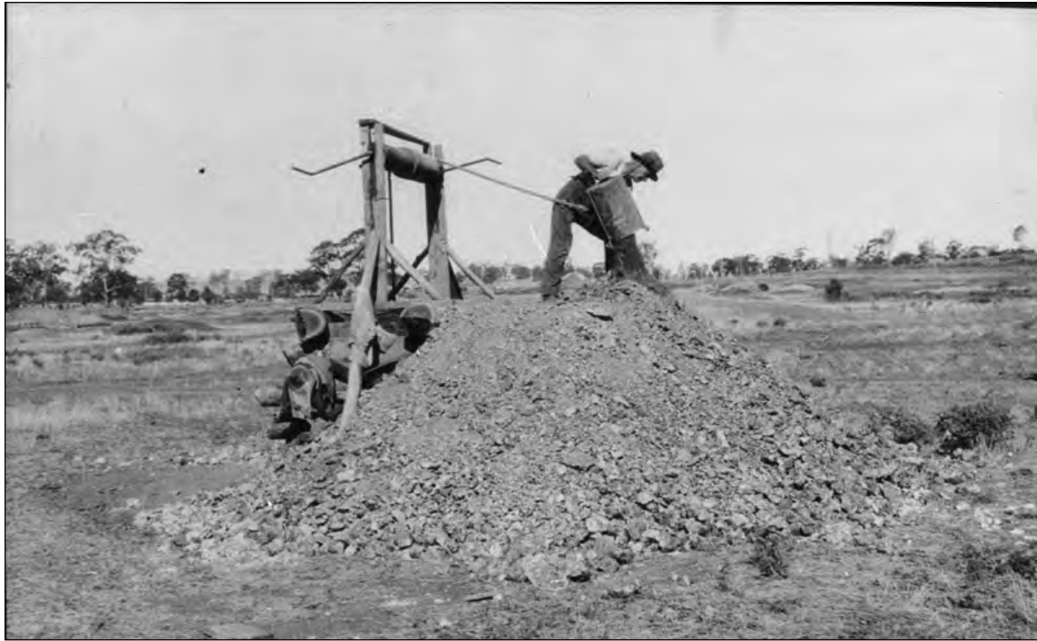
Plate 2: Mine workings at Temora, date unknown
