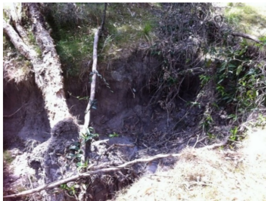
Plate 2: Active erosion point on tributary to main creek
