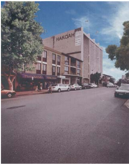
EXISTING – 61 – 79 Hall Street
