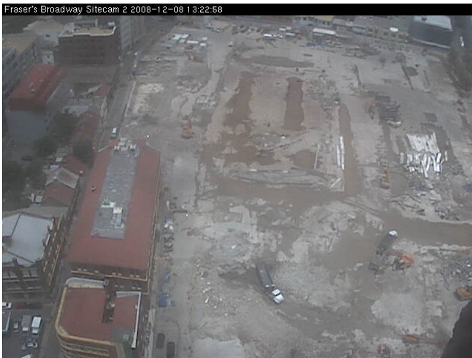
Figure 4 - Aerial view of the site showing extent of demolition works undertaken to date
