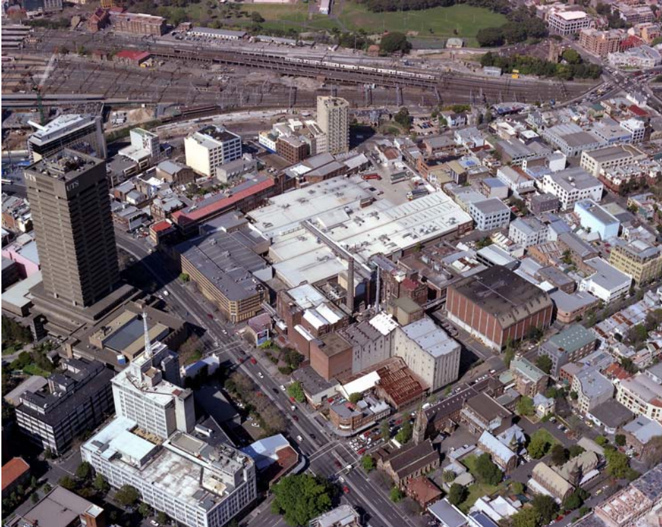
Figure 3 – Aerial view of the site prior to commencement of demolition works
