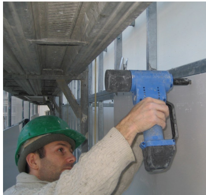
2. Riveting PVC on metal structure
