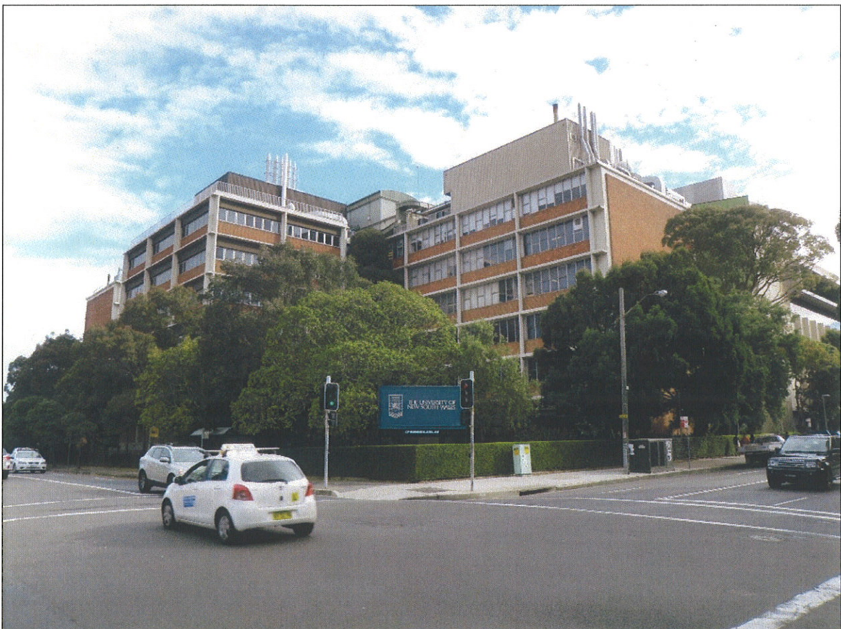
Figure 4 – View of the existing WWB from the corner of Botany and High Streets
