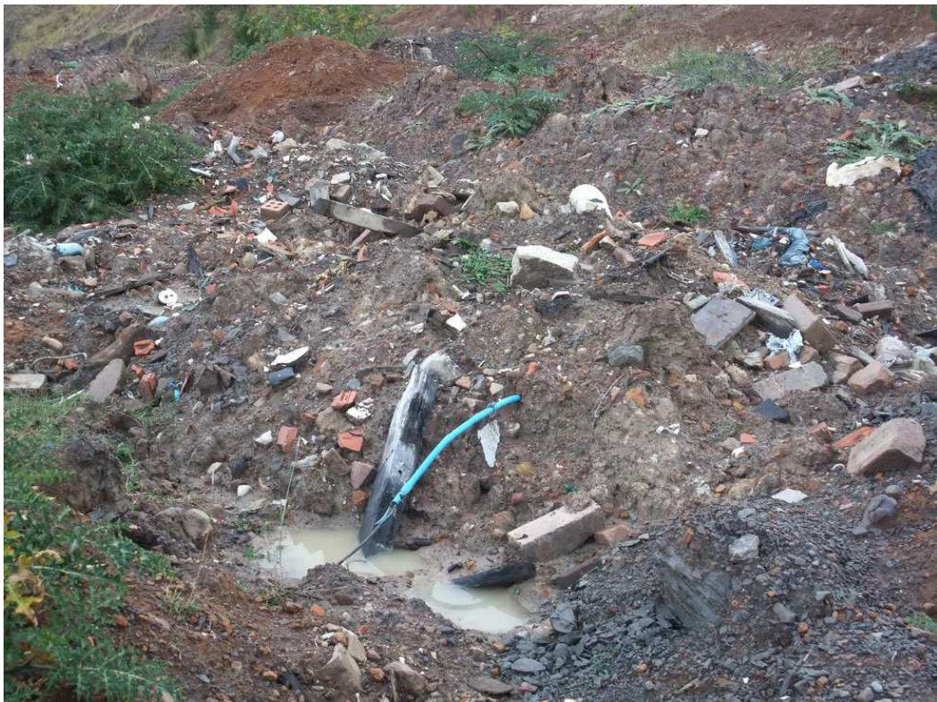
Figure 3: The current state of the site and evidence of unauthorised fill (photo courtesy Penrith City Council)
