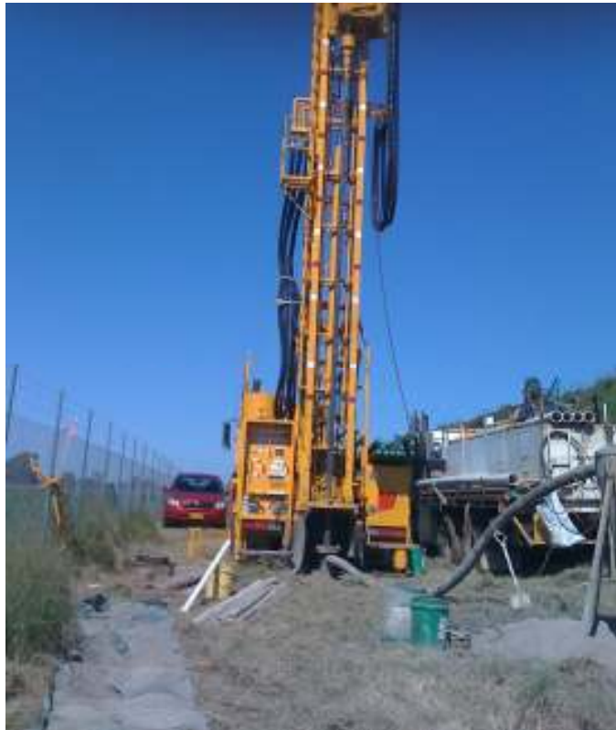
Drilling NE Piezometer PLATE 2
