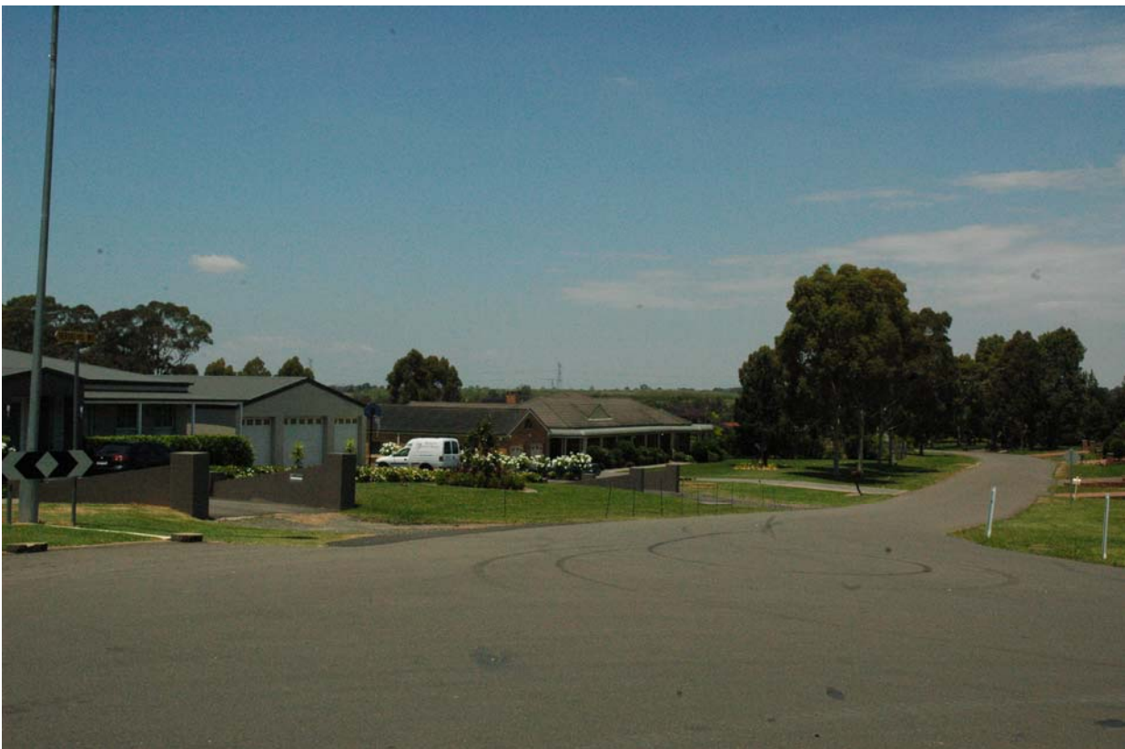
Montage 4: Intersection of Verdelho Way & Wentworth Road – View After 6 Months
