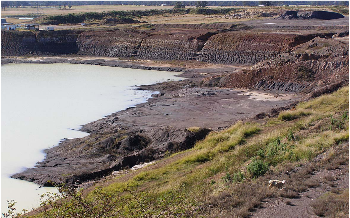
Plate 5: View from the western bundwall with the equipment compound on the left
