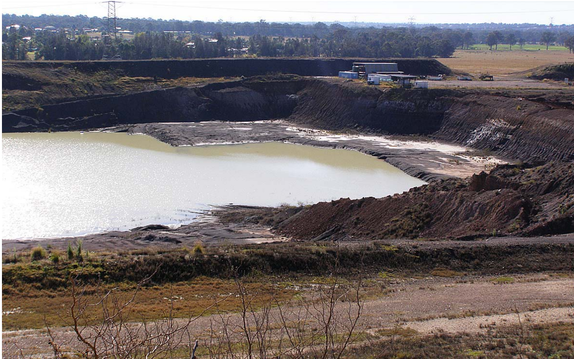
Plate 3: Looking towards the equipment compound from the cut-back in the western bundwall
