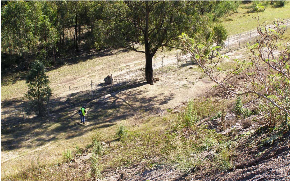
Plate 7: Erosion feature along the western perimeter track in the north-western corner
