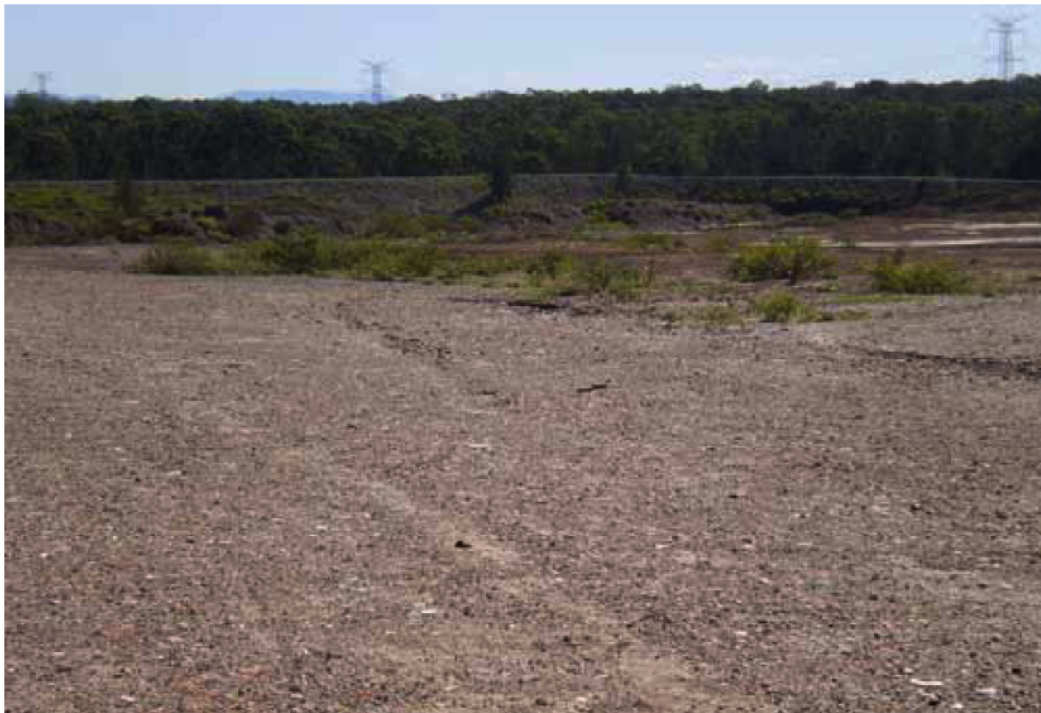
Photo 4: General view of the bund wall north-west of the void
