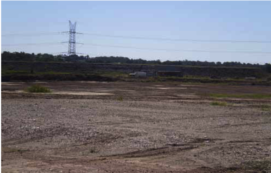
Photo 3: General view of the north-western bund wall
