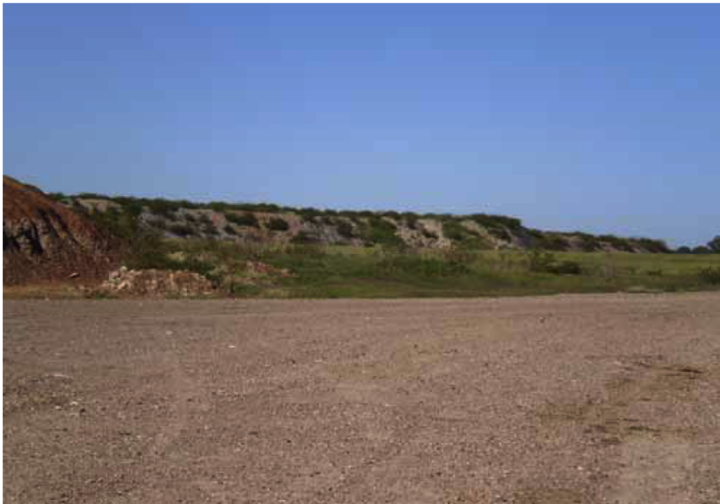
Photo 2: General view of the south-eastern bund wall
