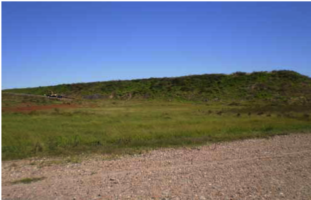
Photo 1: General view of the south-western bund wall
