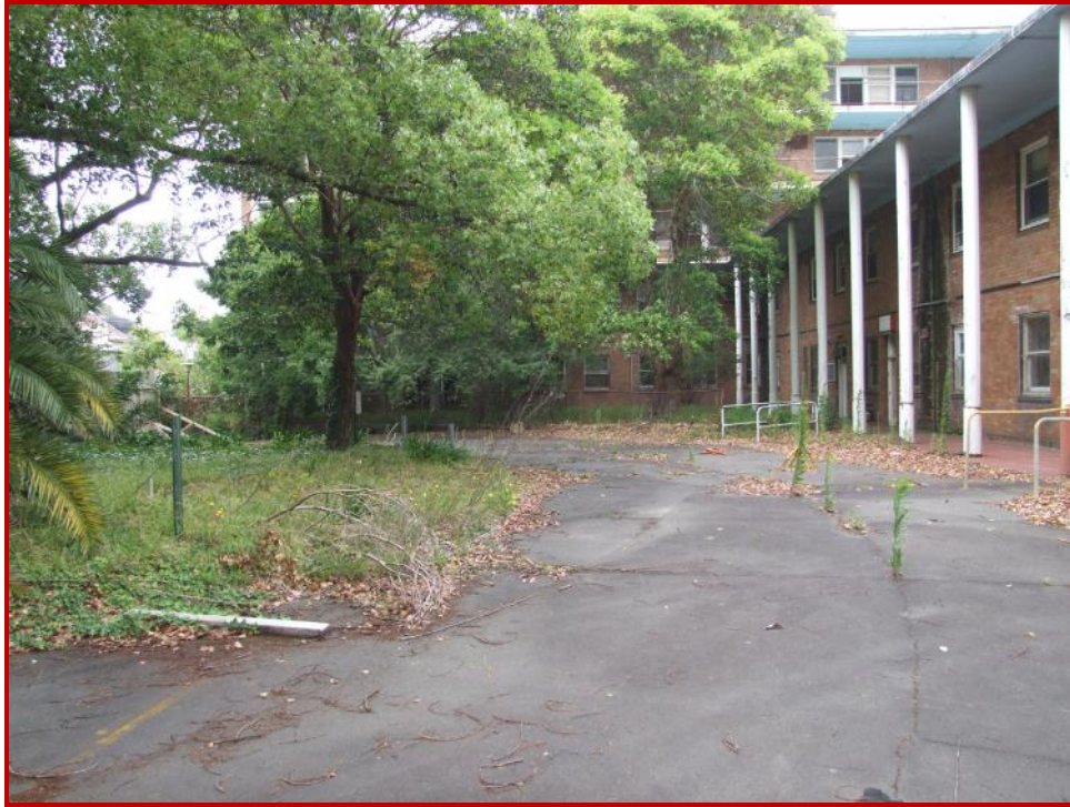
Figure 20. The eastern portion of the subject area, looking south. This area has remained largely unchanged since the hospital's construction in the 1940s.
