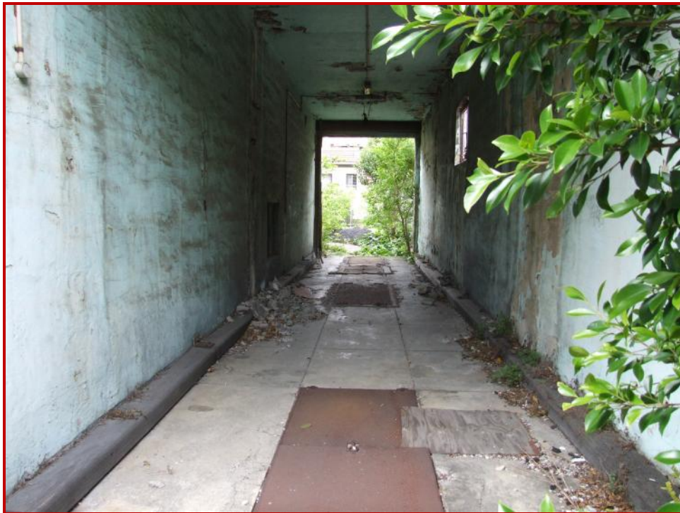
Figure 19. The southwestern corner of the subject area, looking south. Note the service areas for vehicles running through the centre of the thoroughway. Inspection suggests excavation to significant depths in these areas.
