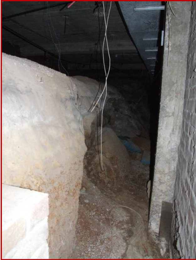
Figure 22. Photograph of an intact soil profile in the basement of the main hospital building, looking south. Note the dark black/brown topsoil overlying a thin pale sand unit over orange/red brown clay. The deposit extended to the south for several metres.
