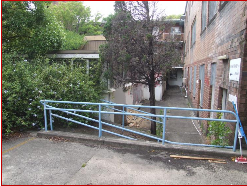
Figure 18. The northwestern portion of the subject area, looking east. Note the excavation of this area to create a level building site.
