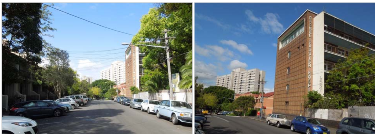
Figure 10 – View along Pitt Street Looking South
