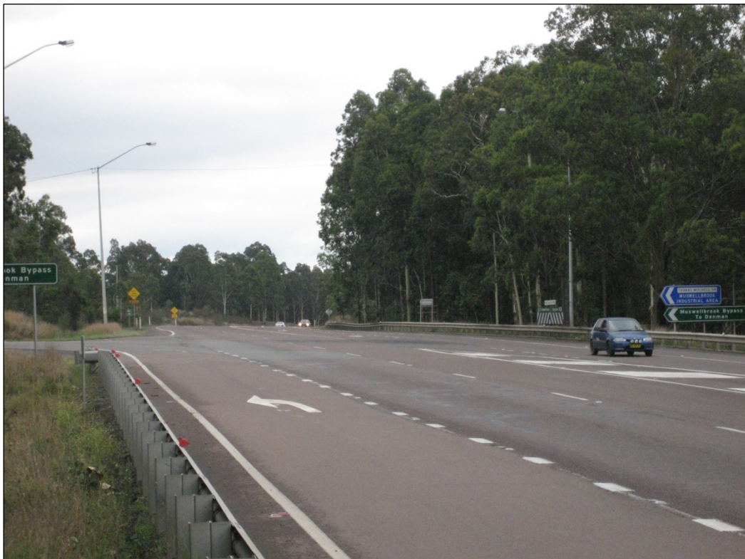
Plate 2 New England Highway / Thomas Mitchell Drive Intersection (looking north along the New England Highway)
