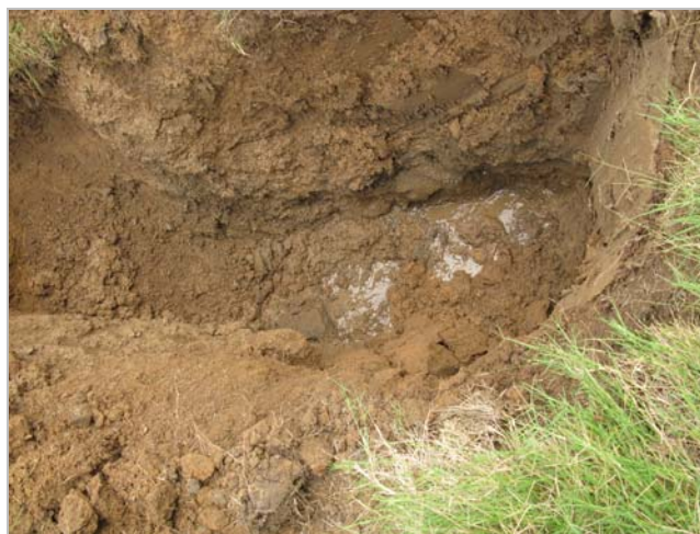
STP1: Showing Groundwater Seepage
