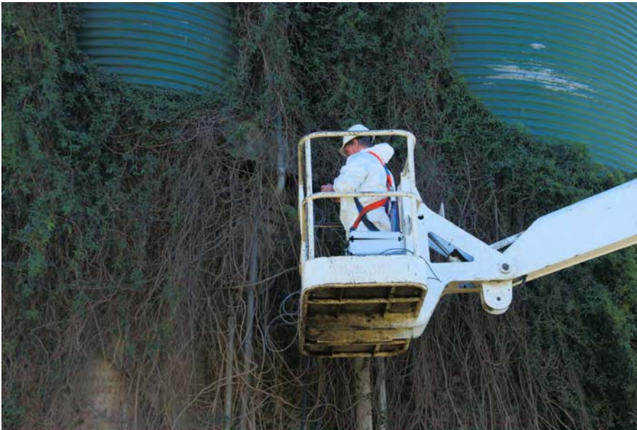
Figure 3: The three sensors were set up on top of the brickwork at the narrow end of the tank stand at a location where maximum movement was expected in the first mode vibration.
