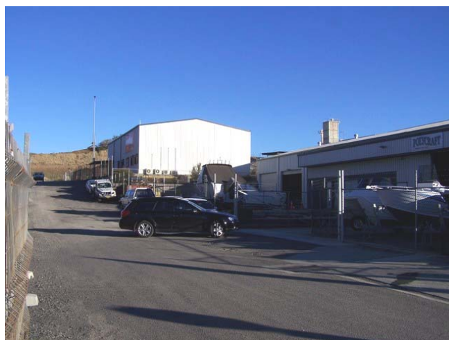
Fig 3: The access handle showing the ROW from the Princes Highway (looking south)
