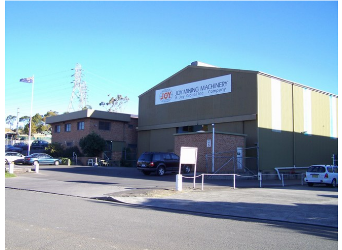
Fig 5: Joy Mining Machinery to the south east of the subject site
