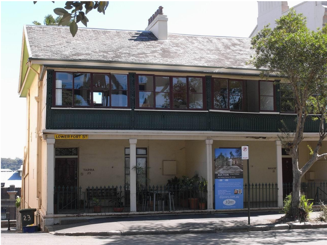
Figure 5: The front elevation of the subject semi-detached houses, Nos 21 (left) and 23 Lower Fort Street. Parbury Lane is on the left.
