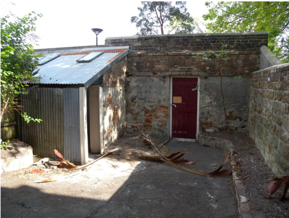
Figure 8: View of the rear of the property showing the original privy closet, evidence of skillion roof and access gate in rear boundary wall.
