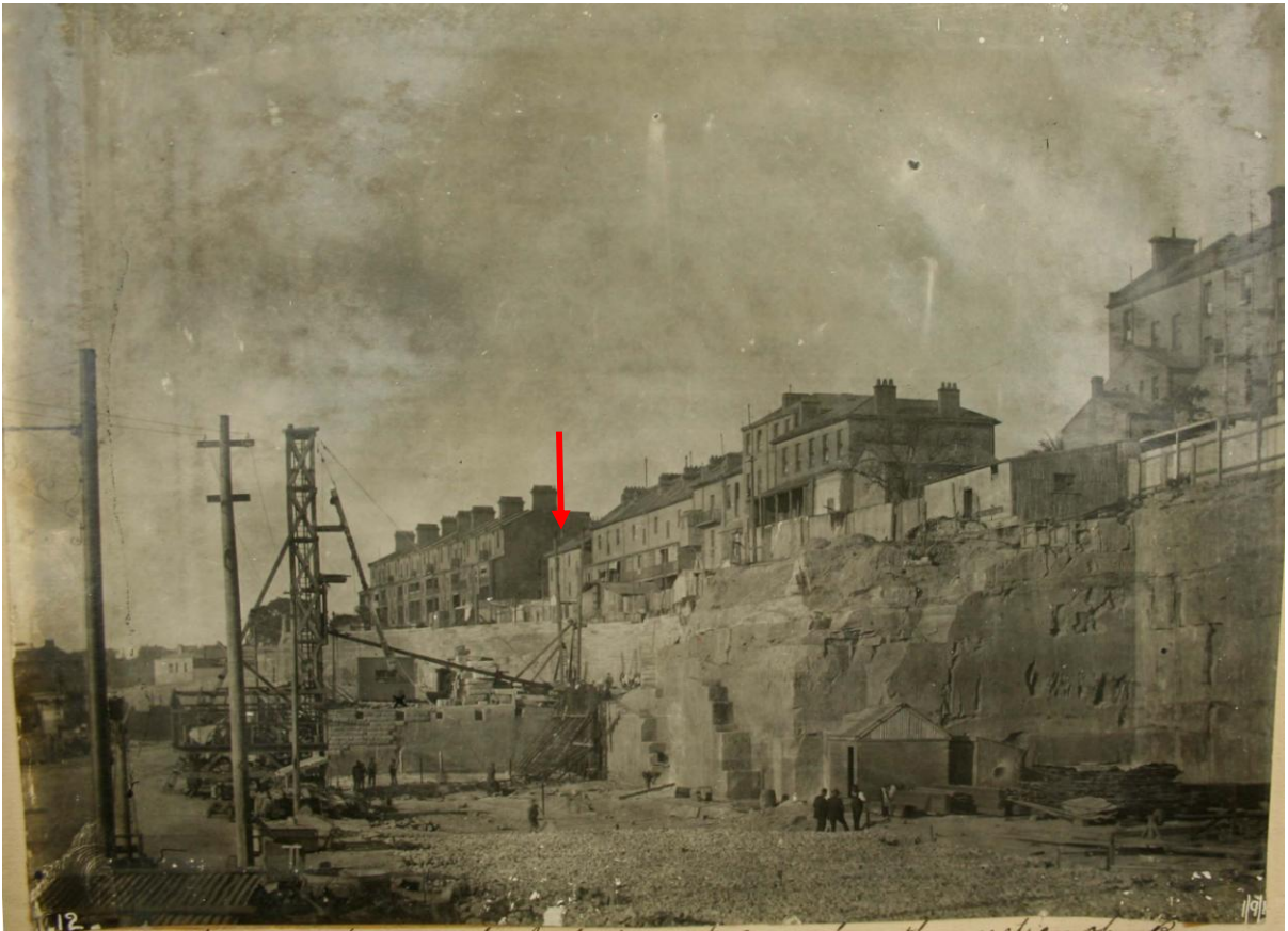
Figure 20: 1916 view from the harbour during the construction of Hickson Road and Pottinger Street and the new wharves, showing the western elevations of the houses in Lower Fort Street. The subject house is indicated, with Milton Terrace to the left and Linsley Terrace to the right. Stables or other ancillary buildings are no longer visible to the rear of the property. Note the mix of skylights and dormer windows to the rear roof planes and the later addition 'clip-on' to 35 Lower Fort Street.
