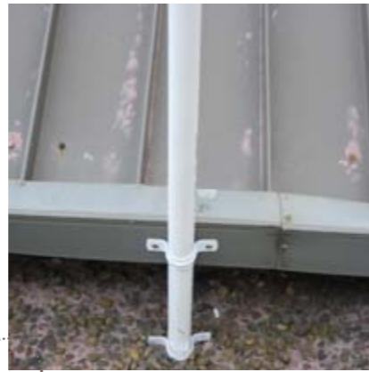
Height poles affixed to existing structure
