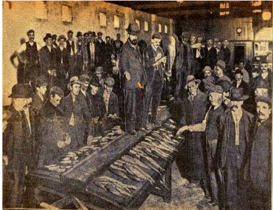
The only known view of the interior of the Redfern Street Fish Exchange (SMH 2 February 1909)
