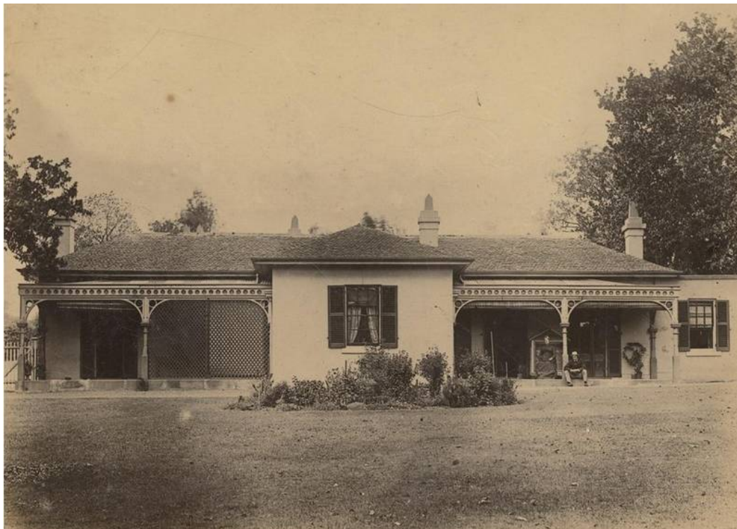
Figure 11: Government Cottage, Carter's Barracks, Fosbery photo, SPF 360.
