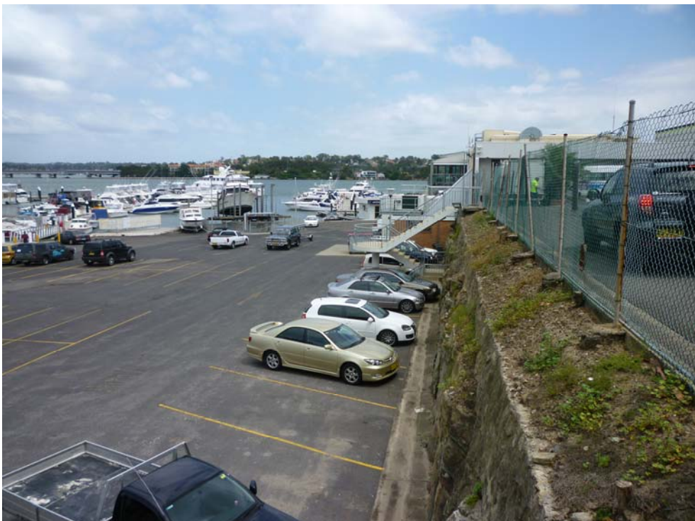
Figure 4: Retaining wall between upper and lower car parking levels
