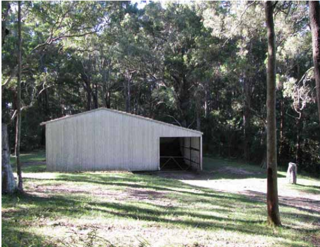
Figure 10: Proposed potable water treatment site: existing shed
