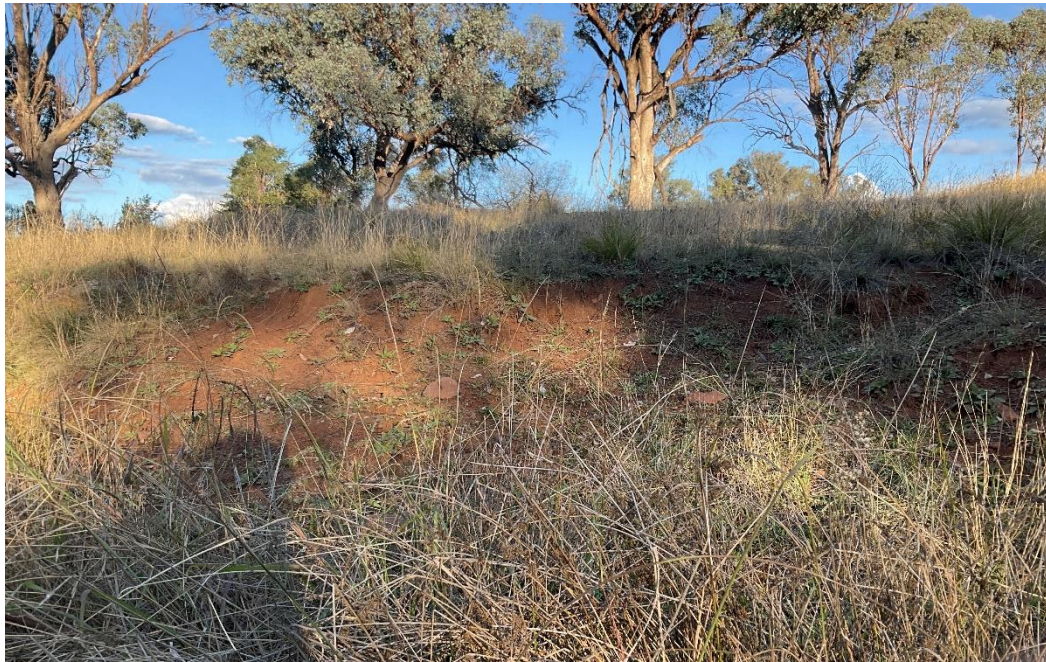
Plate 37 – Erosion Stabilisation Monitoring
