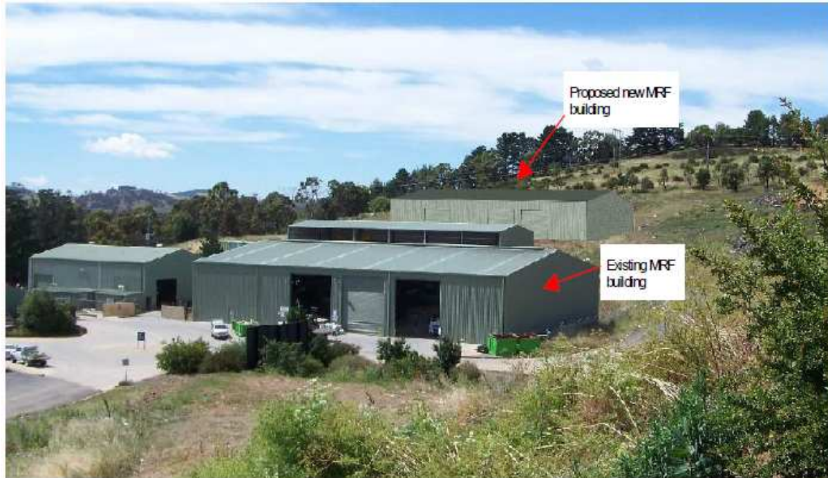
New materials recycling facility at Ophir Rd site
