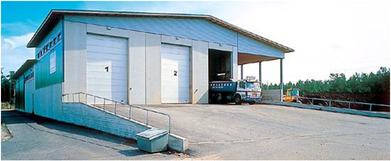
Photo C.1-1 Enclosed tunnel composting plant (overseas example)
