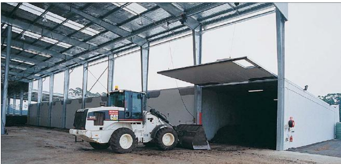
Photo C.1-4 Unloading of compost from tunnels at Remondis Plant, Port Macquarie
