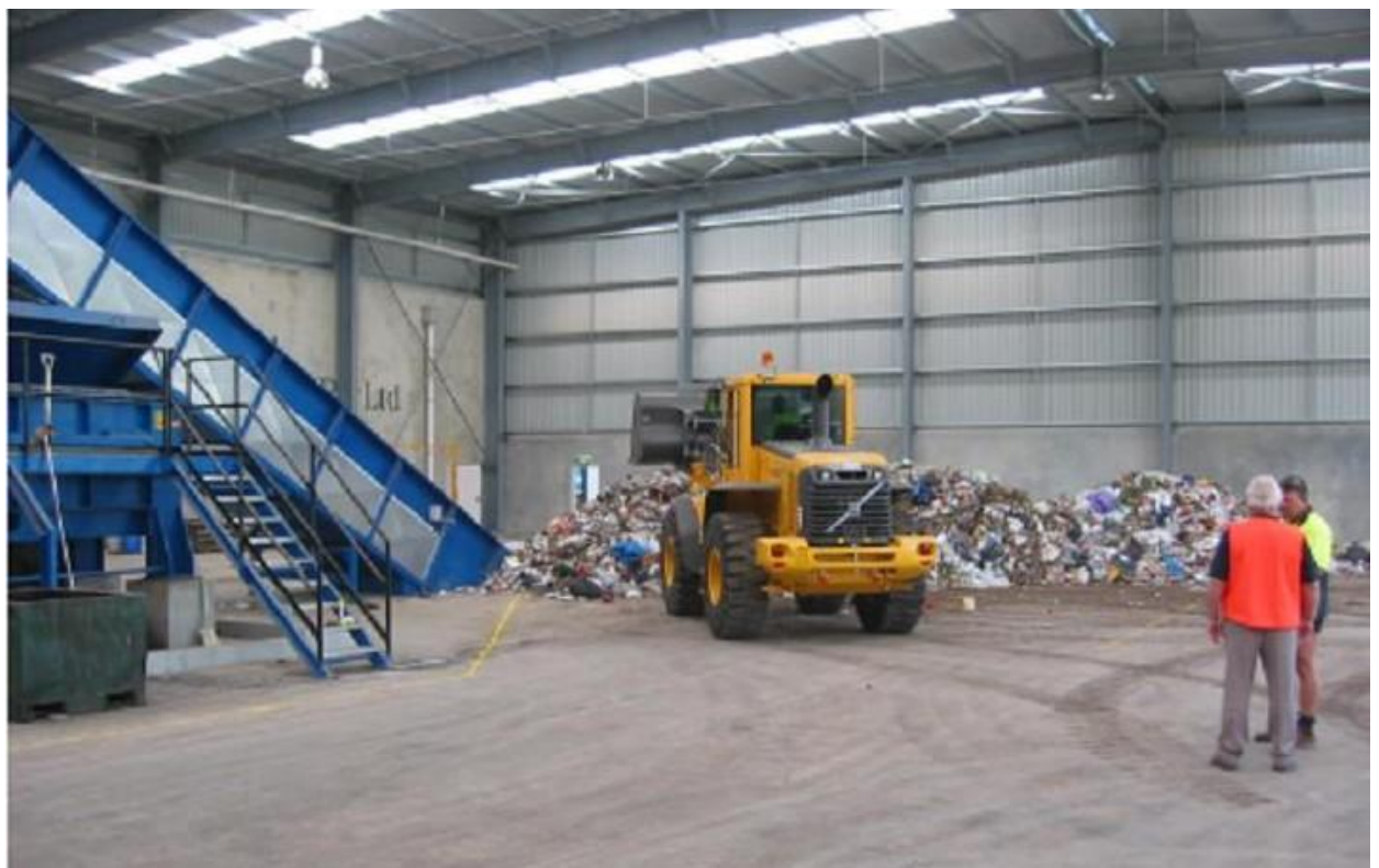
Photo B.2-10 Direct unload onto tipping floor for transfer by conveyor to baling system (example)
