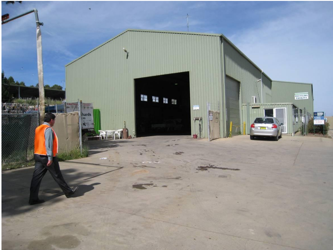
Photo B.1-2 Existing truck storage building and MRF
