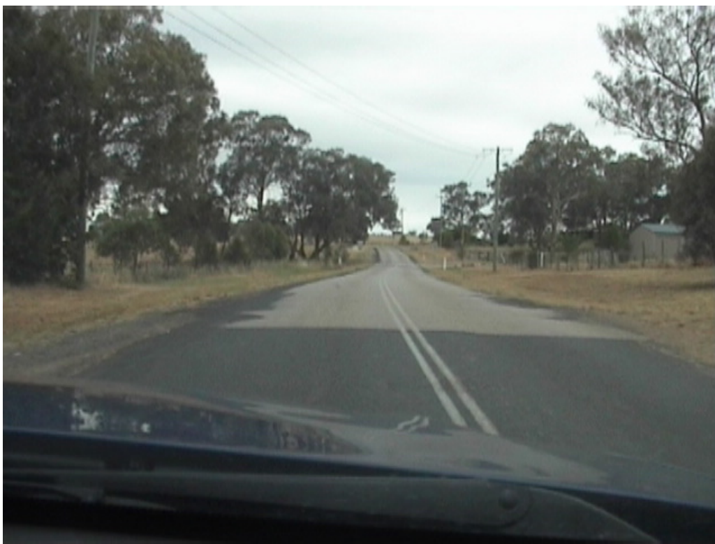
23 – Deficiency Log Item 16 Approx. 100m south of the 50/100 speed zone change the pavement narrows and is extenuated by different pavement colour and textures. Advance warning “Road Narrows” signs (W4-3) may be appropriate under these circumstances.
