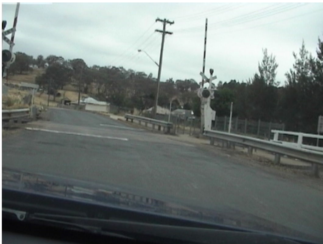
14 – Deficiency Log Item 9
