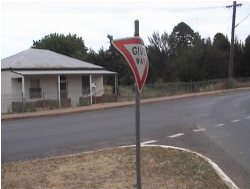
22 – Deficiency Log Item 13
