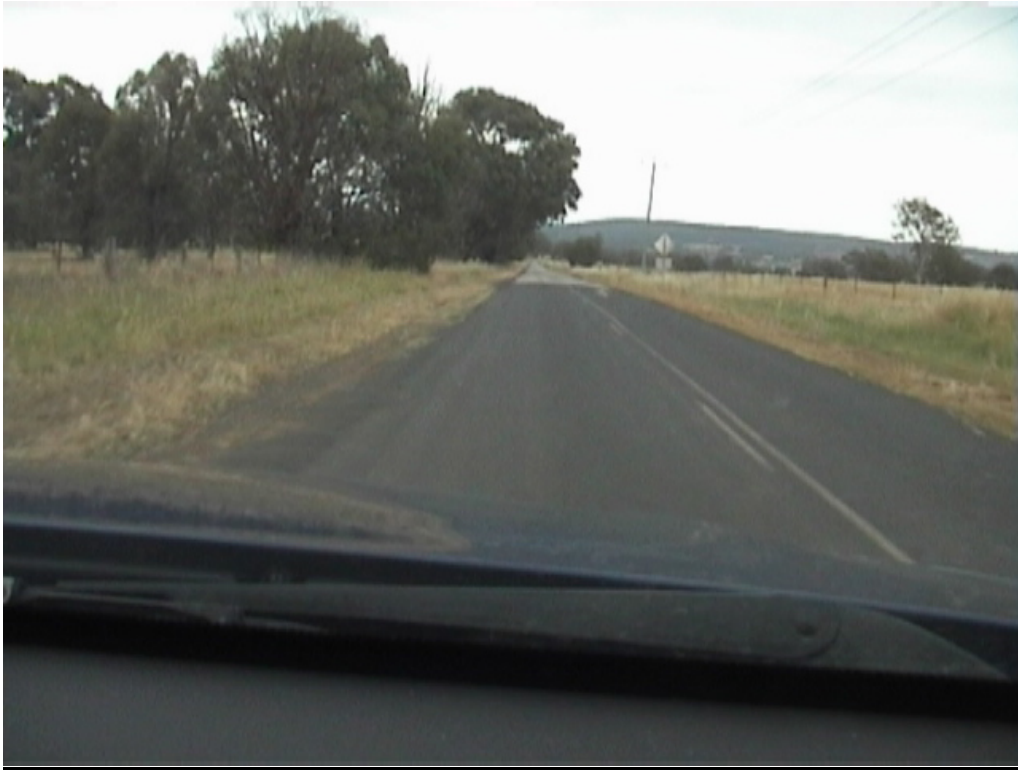
3 - Deficiency Log Item 1
