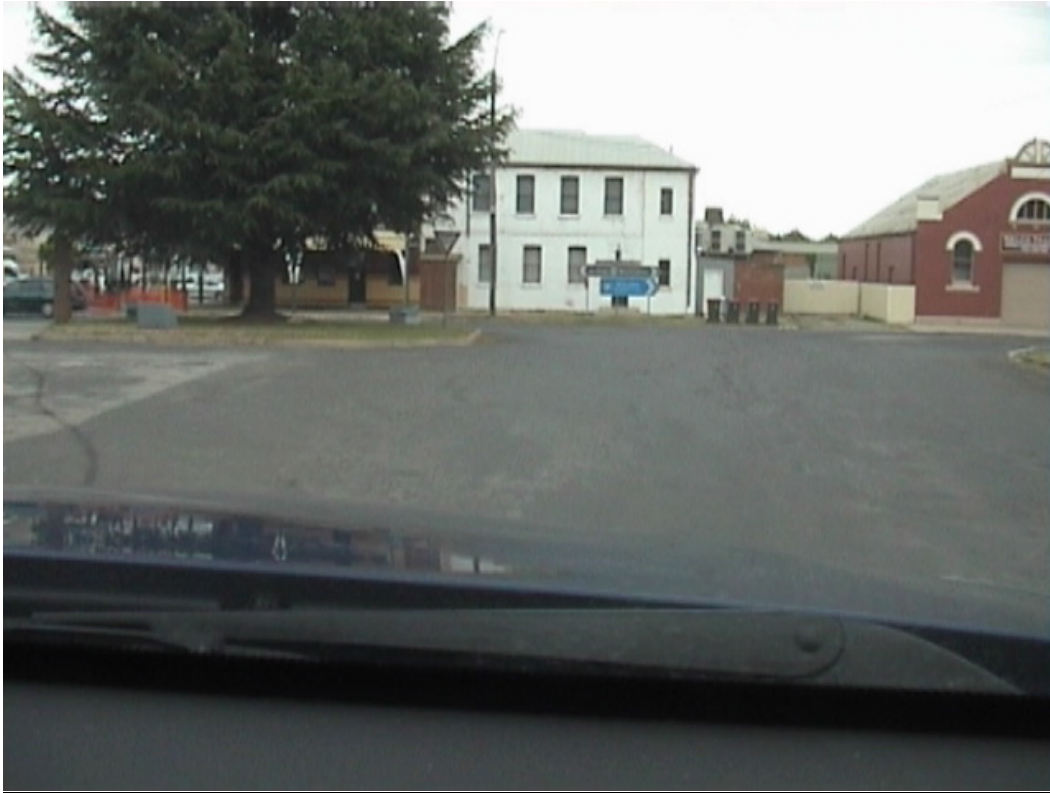
11 – Deficiency Log Item 8 Located approx. 30m to the east of Watson Road (Mitchell Highway) is a vehicle access to the car park servicing the Railway Station Library and Bus Stop. At this point there is an expansive area of uncontrolled pavement and it was observed eastbound vehicles (including Buses) travelled in the opposing traffic flow lane to access the site. The road configuration of this access is considered hazardous.
