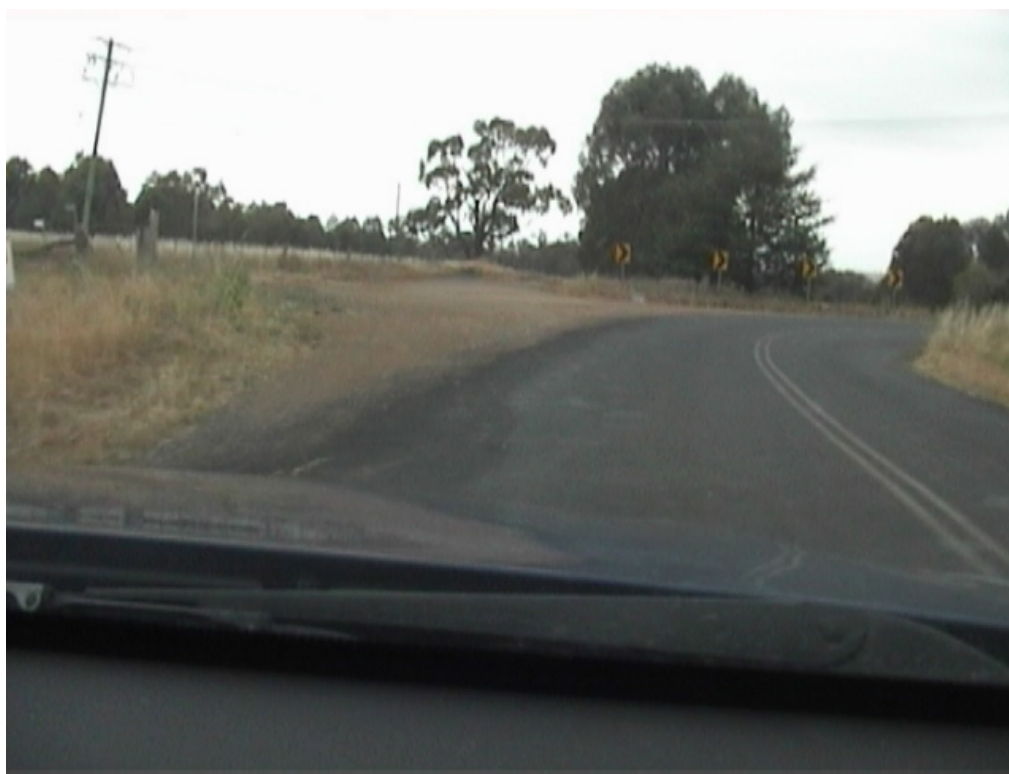
32 – Deficiency Log Item 19
