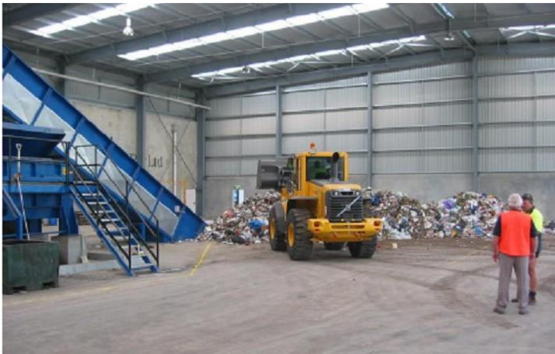
Photo 5-2 Direct unload onto tipping floor for transfer by conveyor to a baling system
