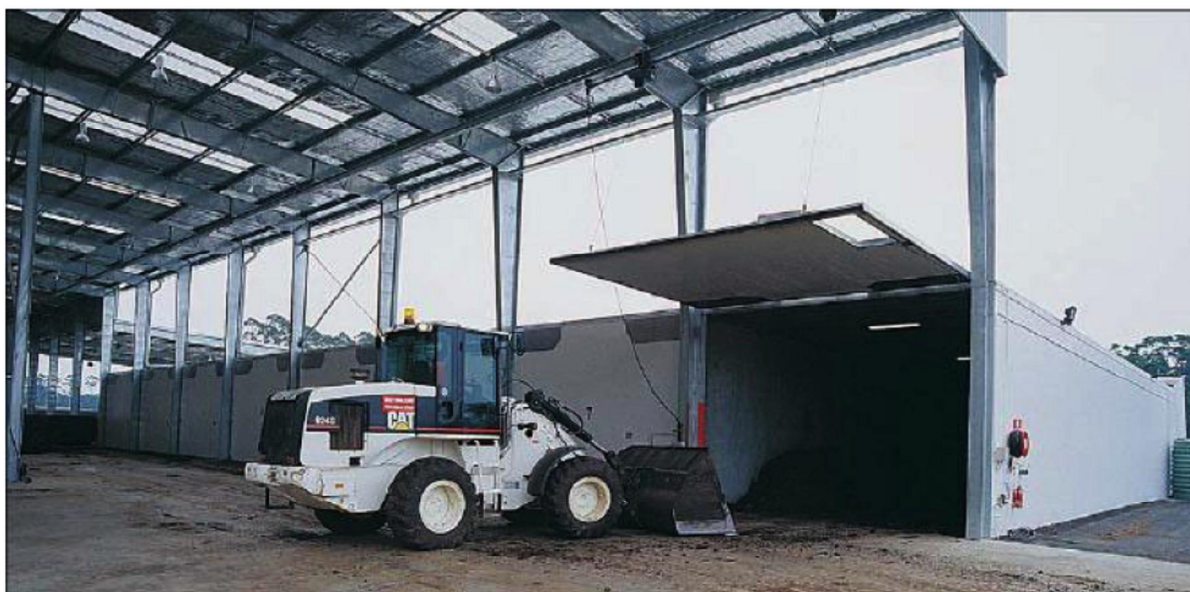
Photo 6-6 Unloading of compost from tunnels
