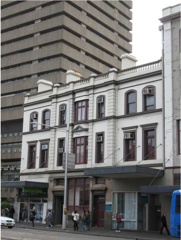
Figure 4 The Terraces (CB08) with the edge of the Bon Marche building visible on the right. (Source: GML 2008)
