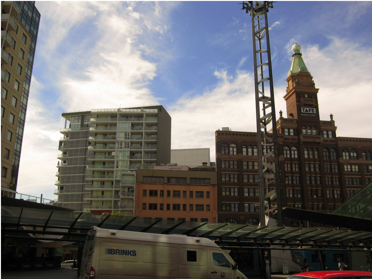
Figure 12 View of the Marcus Clark building from the southern side of Railway Square. The proposed Building 6 would fill the gap in the view between the recent apartment block to the left and the Marcus Clark building to the right. (Source: GML 2009)
