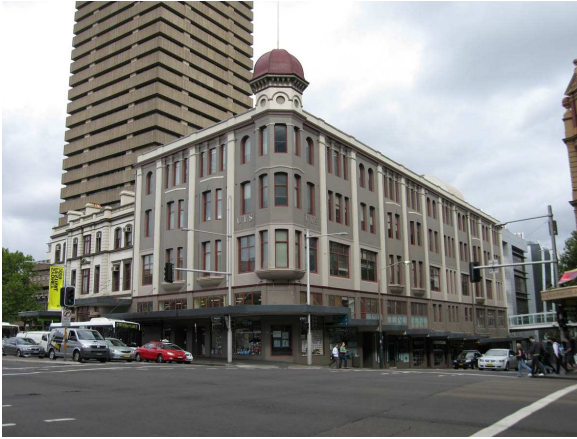
Figure 2 The Bon Marche building (CB03) on the intersection of Broadway and Harris Street. (Source: GML 2009)
