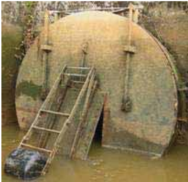
Plate 1. A pipe with an automatic tide floodgate.
