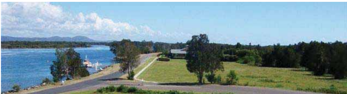
Plate 3.1 View of site looking north towards the tavern
