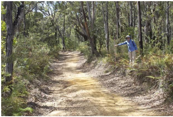
Photograph 5.33 52-3-0313 Bulli Mine Shaft 29 – Access track to Brokers Nose Ridge highlighting the level of erosion along this track.
