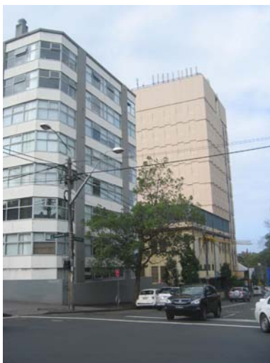
Picture 7 – Development to the immediate north, across Liverpool Street (new building under construction on central site).
