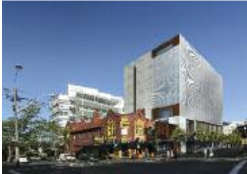
View demonstrating visually solid screen on northern facade
