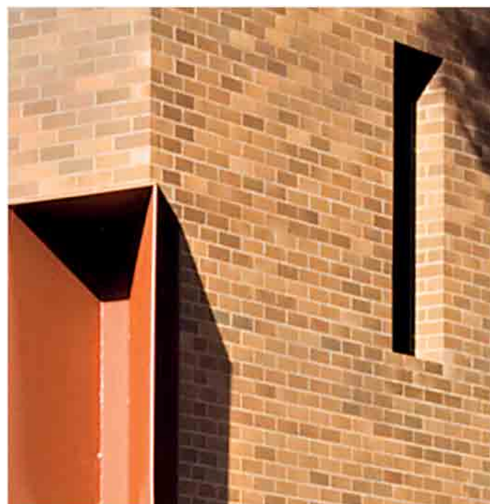
[PSS] PAINTED STEEL STRUCTURE (Colour - Red Oxide)
