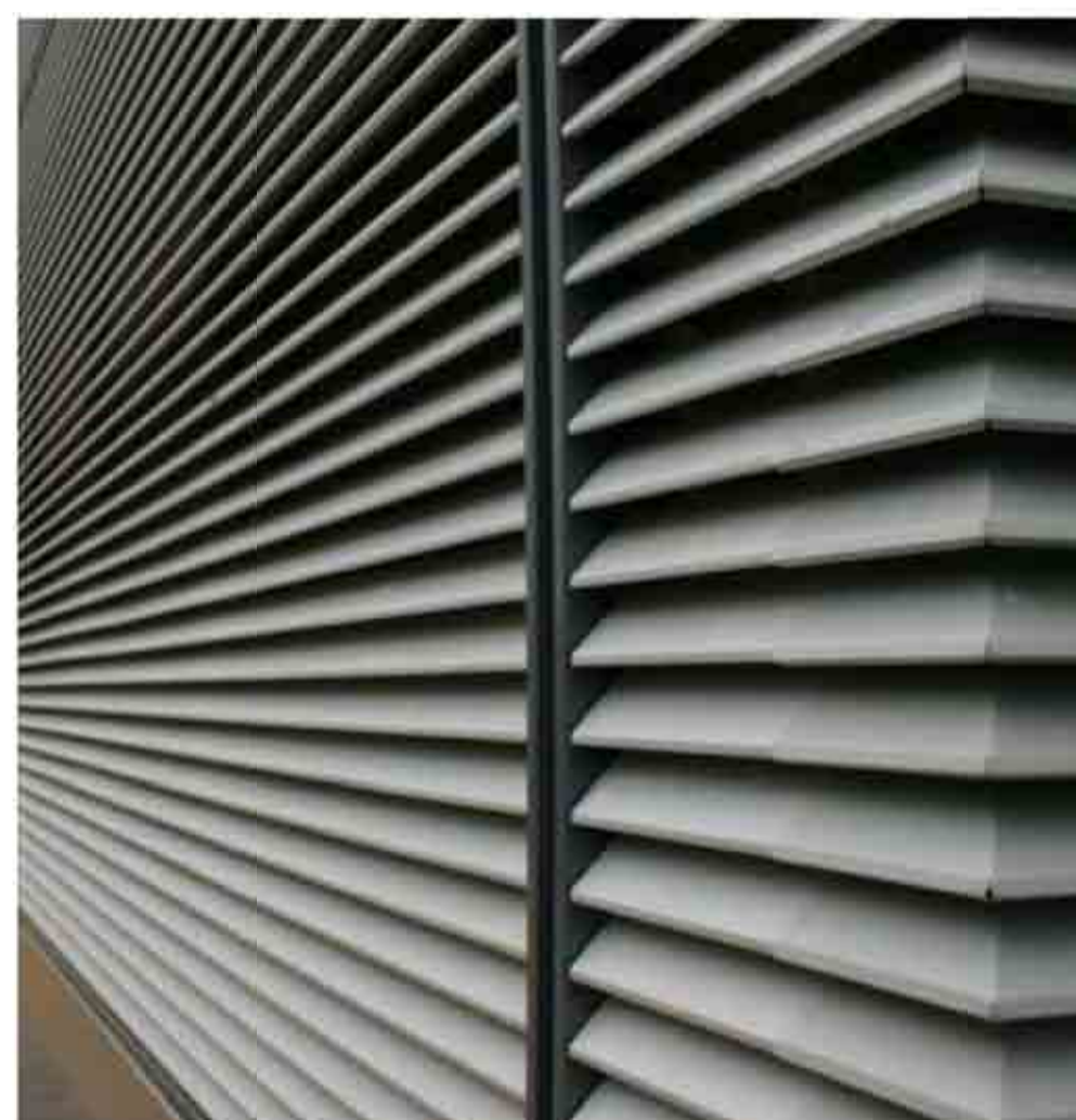
[MLPG] METAL LOUVRE PANELS (Powdercoated finish - Light Grey)
