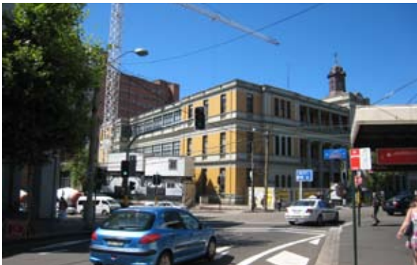
Picture 14 – The original (deLacy) St Vincent's Hospital building, with Cahill Building in background'
