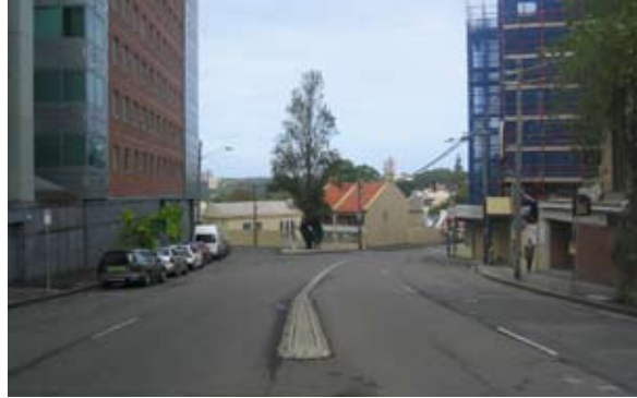
Picture 13 – Burton Street and St Vincent's Hospital O'Brien Building (currently under construction)
