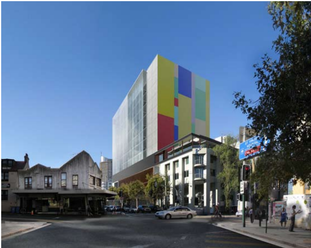
Picture 16 – Looking north-east from the corner of Burton and Victoria Streets (artwork is indicative only - see Section 4.9)
