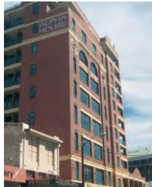
(H) ALPHA HOUSE, KING STREET
