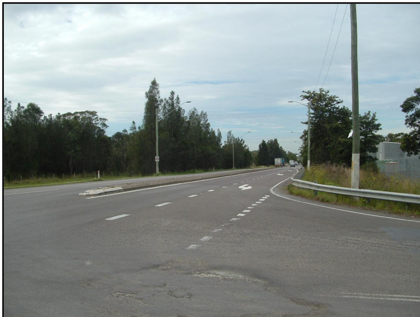
■ Photo 3 – View east along New England Highway at Kyle Street intersection
