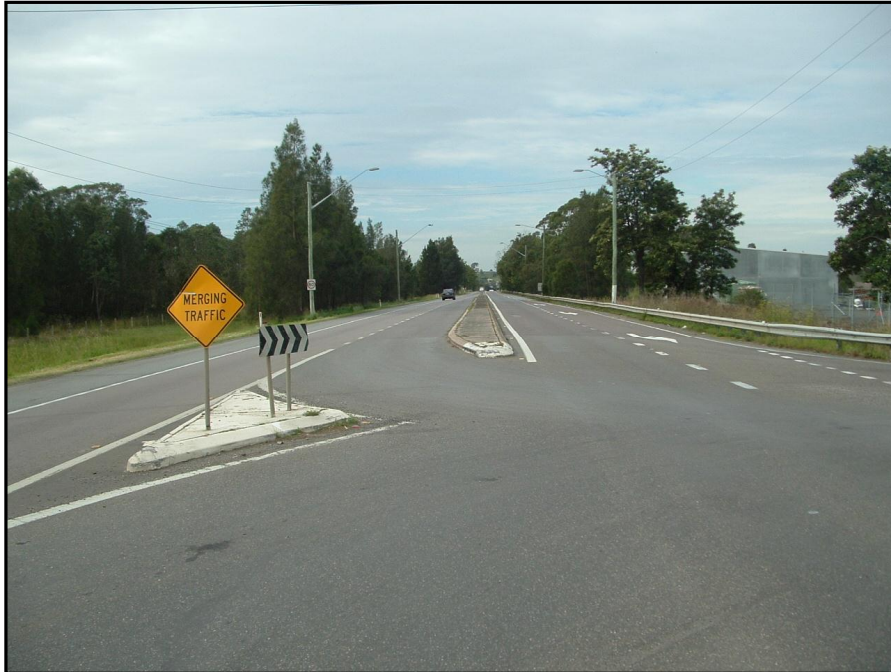
■ Photo 7 View east along New England Highway showing visibility splay for traffic entering Kyle Street.
