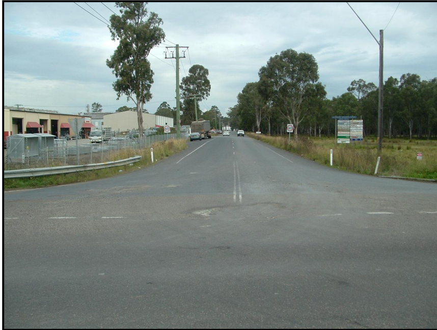
■ Photo 2. View south along Kyle Street showing typical cross section
