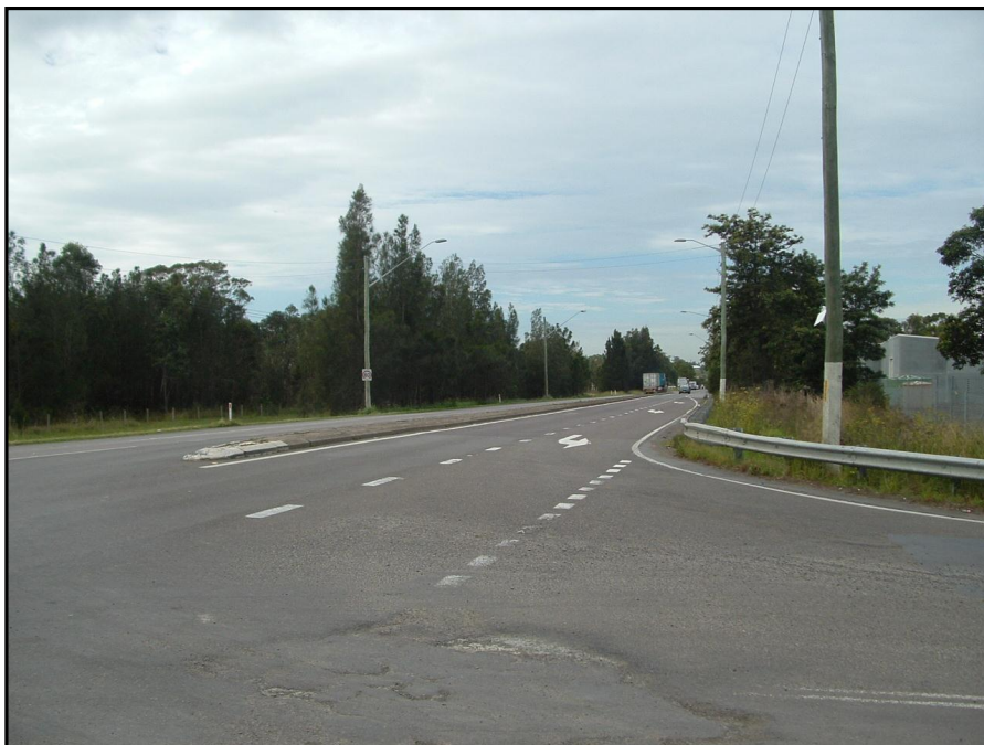
■ Photo 8 View east along New England Highway showing visibility splay for traffic exiting Kyle Street.
