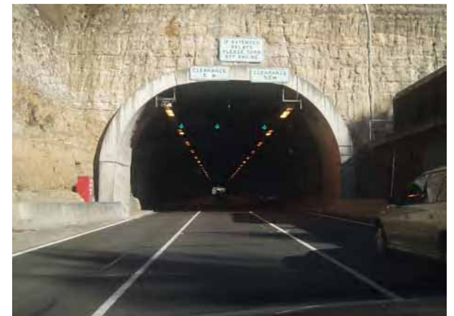
Photo 2.12 Tunnel portal area reveals the local geology
