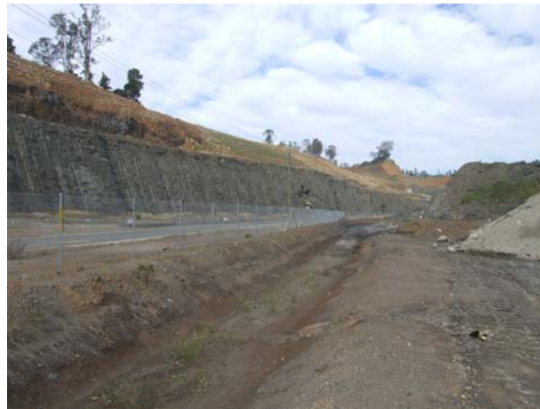
Figure 2.3.3 North-eastern batter looking south
