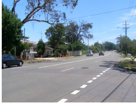
Figure 12 – Marsden Road/ Mobbs Lane intersection
