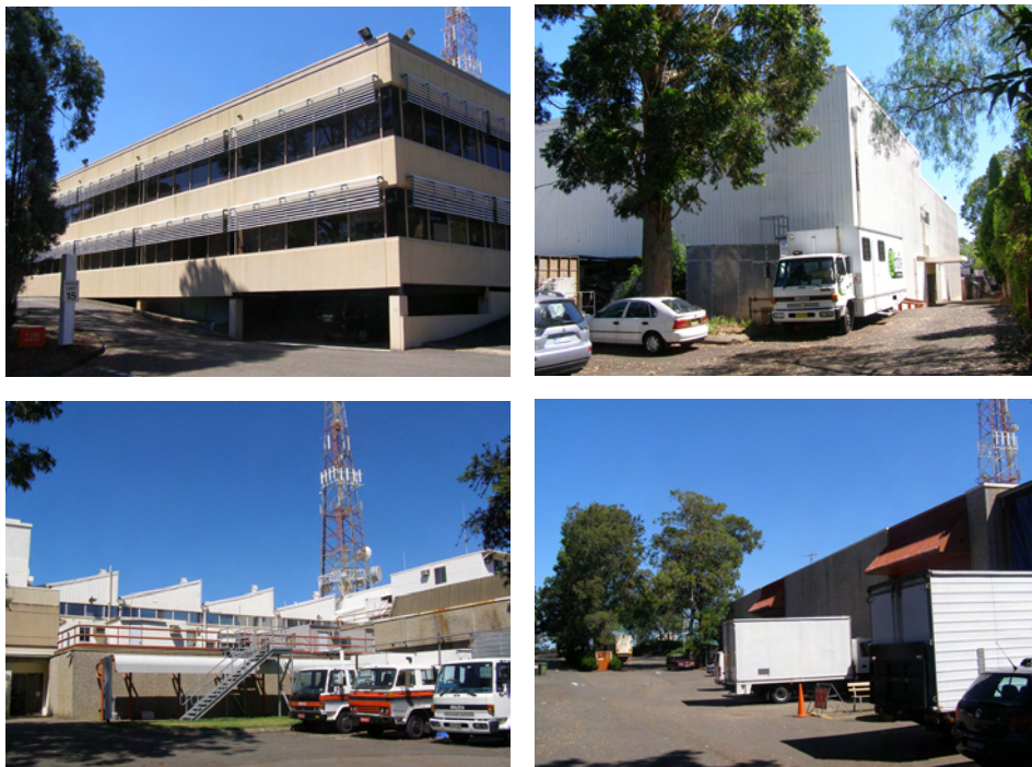
Figure 4 – Television studios and ancillary buildings
