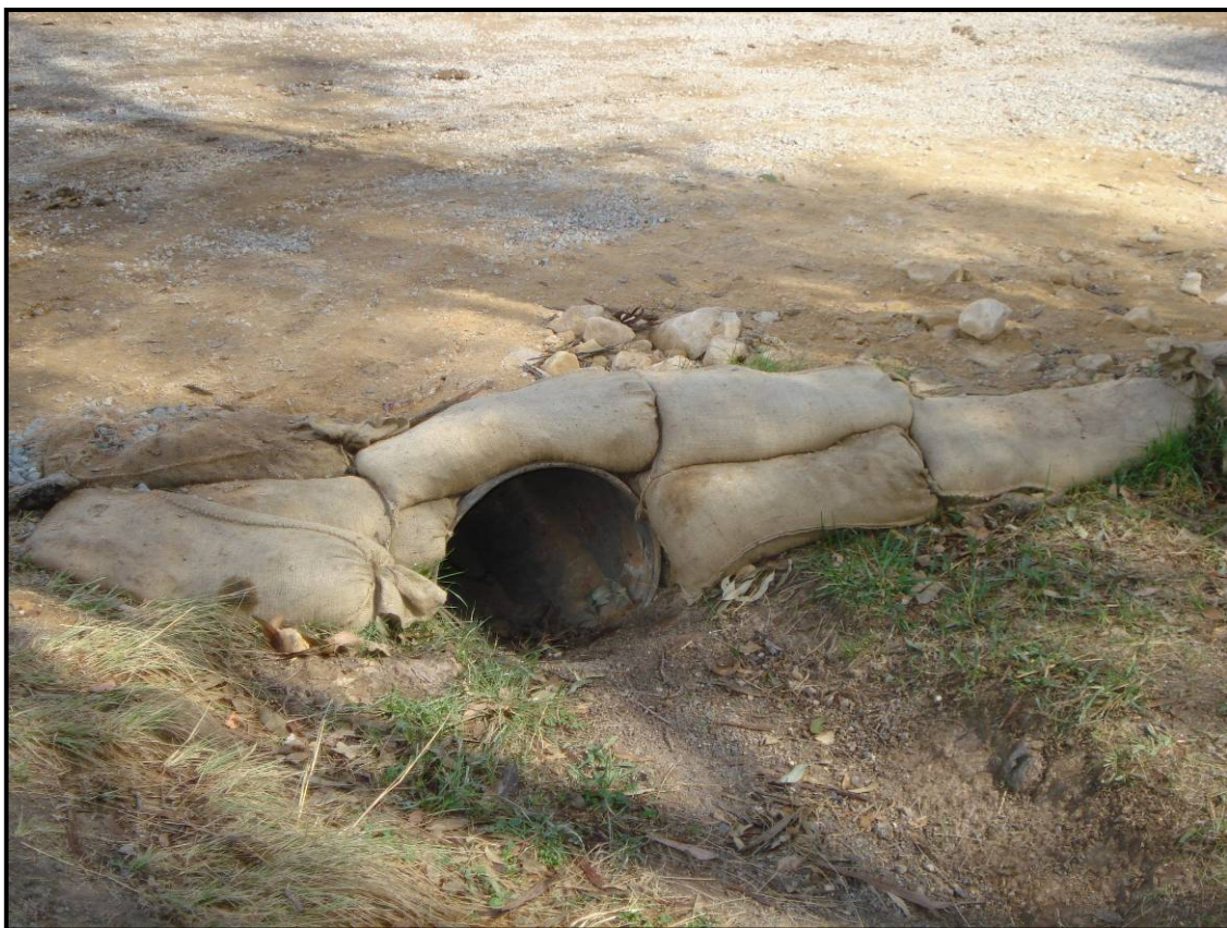
Figure 10 Erosion and Scour Control Structure
