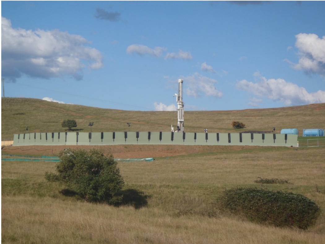
Figure 8 Typical Noise Mitigation Barriers
