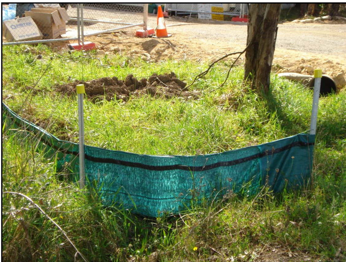
Figure 11 Sedimentation Control Structure
