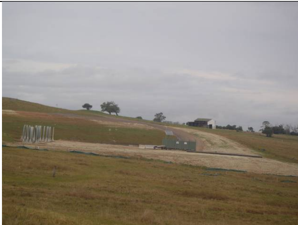
A well site soon after construction has been completed with equipment removed, well infrastructure installed and drill pad temporary rehabilitation installed.
