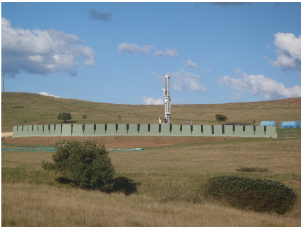
Figure 9 Typical Noise Mitigation Barriers
