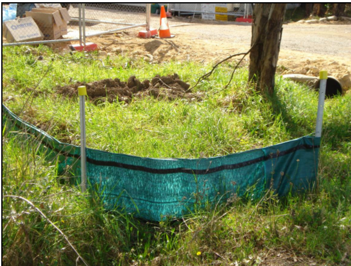
Figure 12 Sedimentation Control Structure
