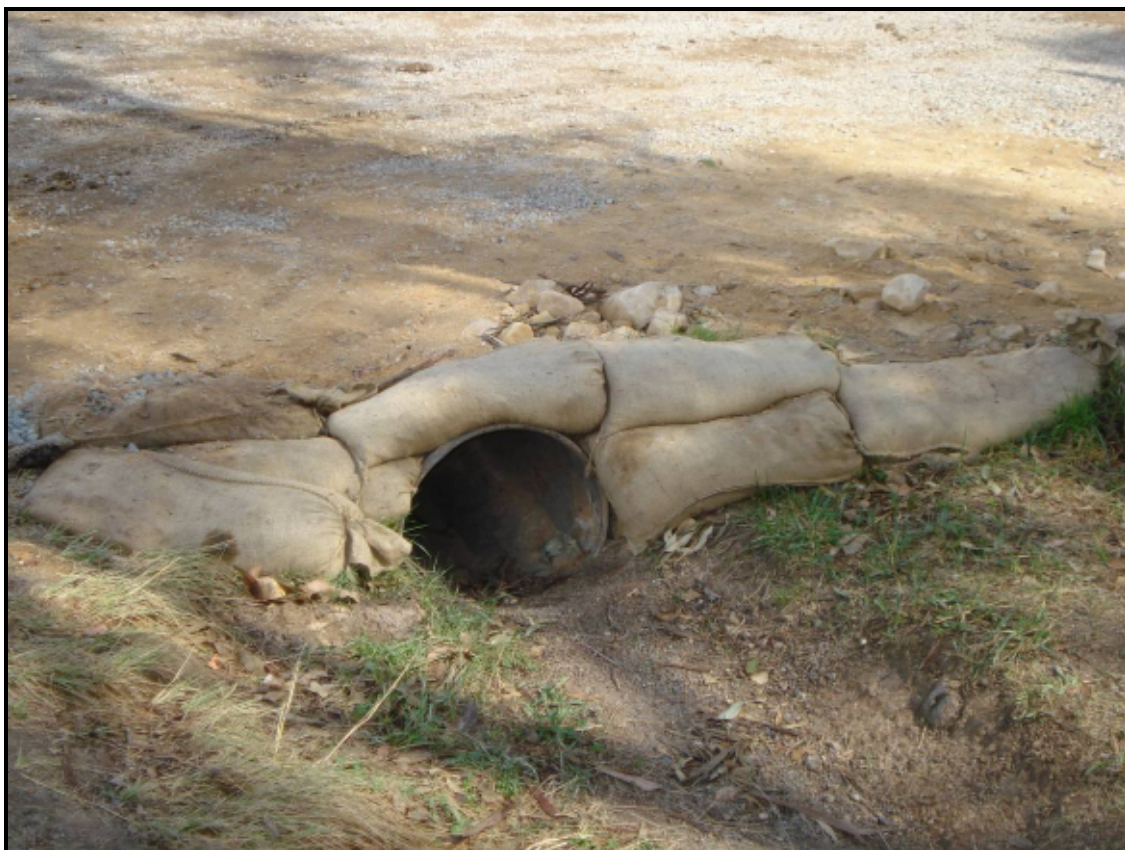
Figure 11 Erosion and Scour Control Structure
