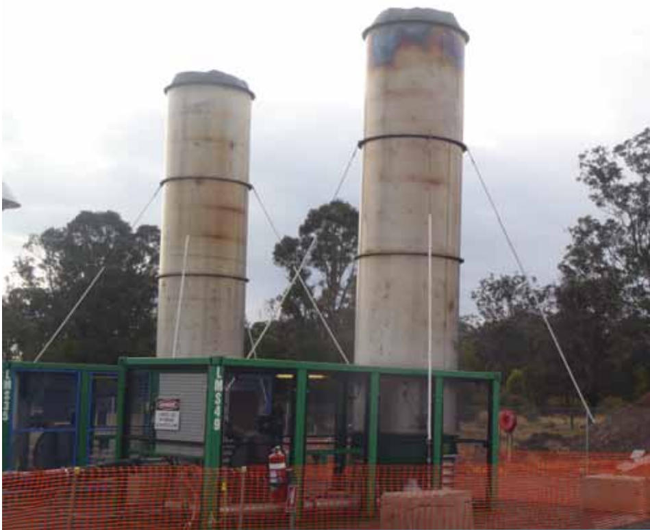
Where possible, gas from mine safety gas drainage holes is piped to methane gas power plants or in some cases is flared in enclosed flare stacks similar to those pictured above.
