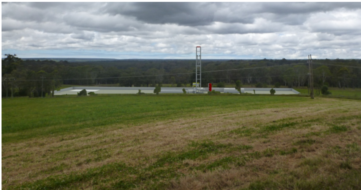
Figure 8 – MSGD Visual Montage - Construction Phase
