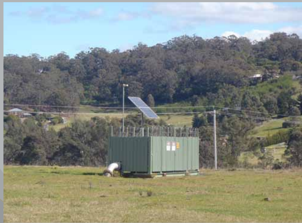
Once drilling activities are completed, the site is backfilled to restore original contour of the land and a small compound is constructed around the wellhead.
