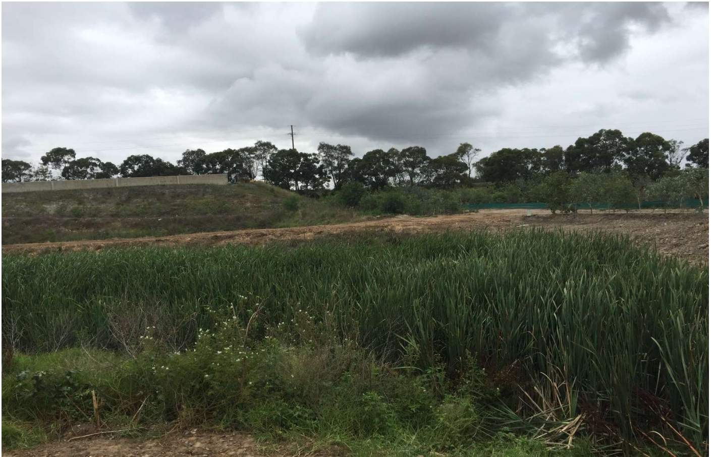
Figure 5 – Reed bed in retention basin.
