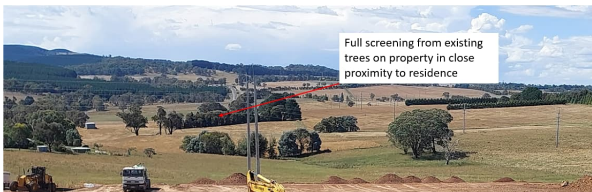
Photo 2 Direct view from Switching station to Newcrest property H2 (looking north)
