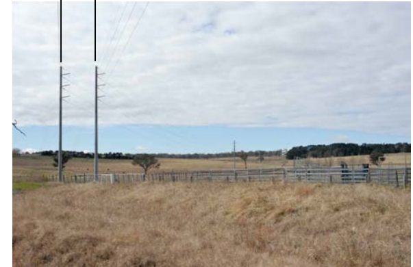
Double circuit 132kV powerline (angle pole structure) at road crossing
