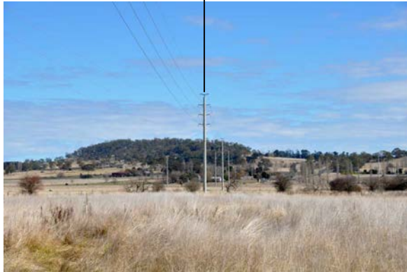
132kV double circuit powerline crossing rural agricultural land
